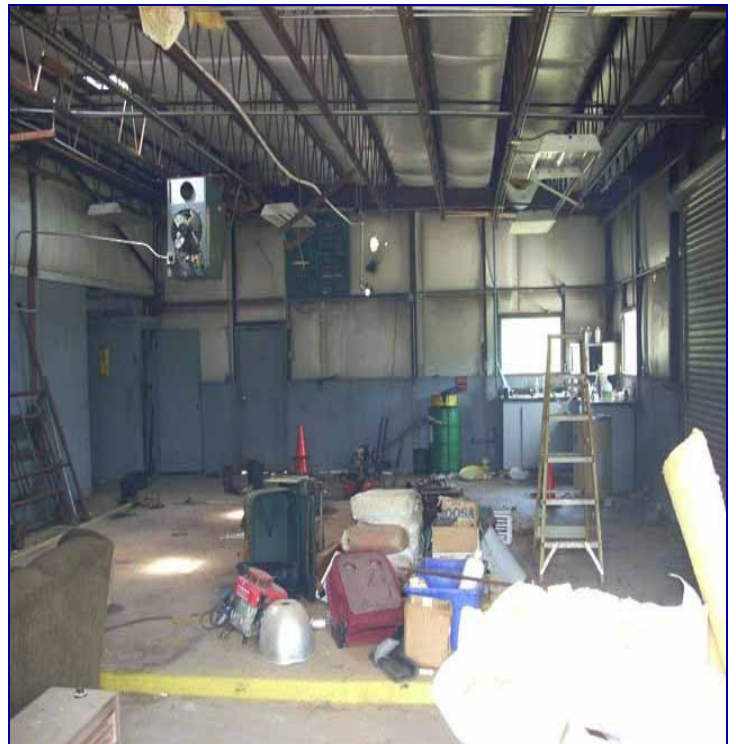
Inside of maintenance facility.
