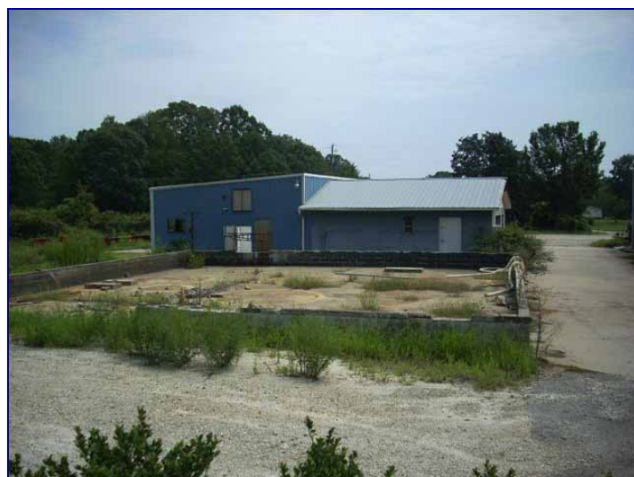
Side view of 2,100 s.f. building.
